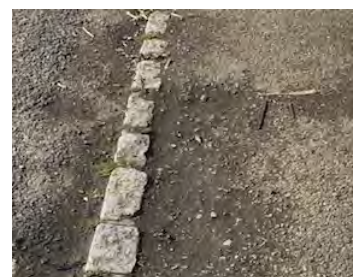
Kerb to footway of granite setts
